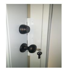
The Pry Shield should be installed on the outside door frame centered to cover the deadbolt and door knob. If the door knob and deadbolt are spaced too far apart, center the Pry Shield with the deadbolt.
