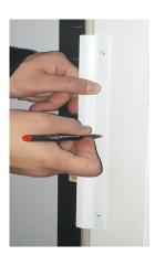
Start by marking the holes you will be pre-drilling with the Pry Shield against the frame.
