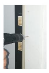
Pre-drill the three marked holes you made in step two with an 11/64" drill bit.
